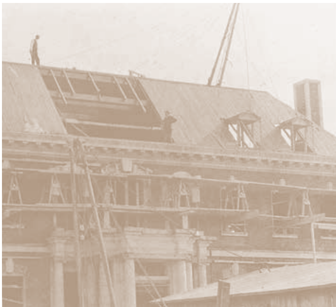
Westbury House construction, 1905.
